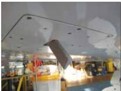
weight down yet maximizing the airframe strength. From the weight perspective he would have preferred to use vinylester instead of polyester to build the wing, because it wets the glass more easily during the layup construction process, resulting in lighter parts. The one-piece wing and one-piece H-spar, at nearly 30 feet long, require a large construction space, but Jean-Dom fabricated this at Brienne, and it was one of the many components he trucked back to his home near Caen.
